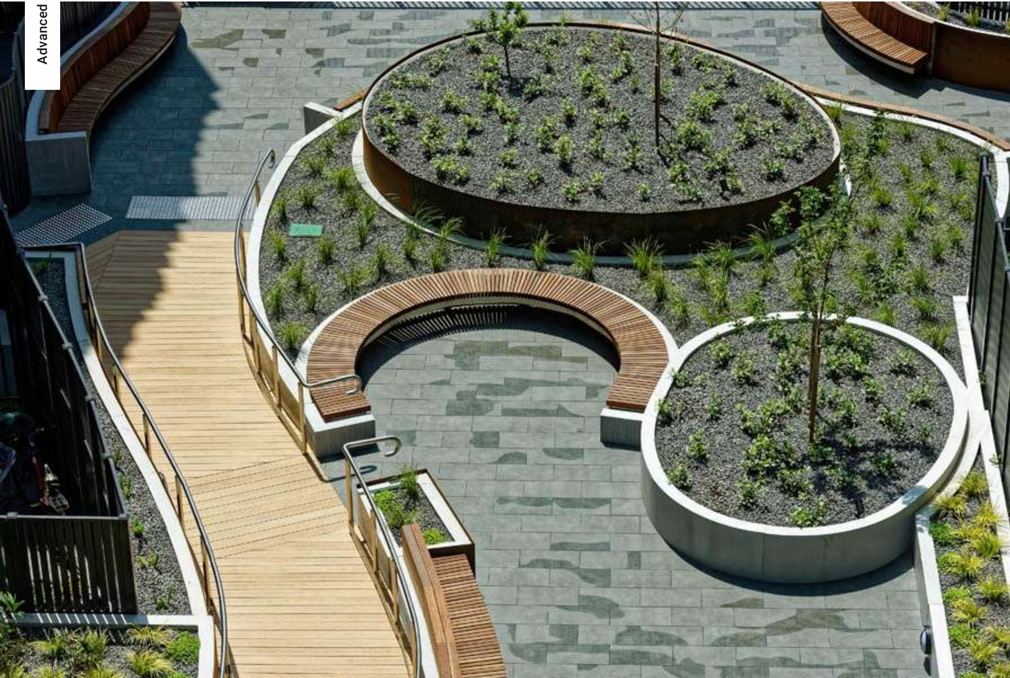
AN EXAMPLE OF THE USE OF CUSTOM GRC PLANTERS WITH INTEGRATED TIMBER SEATING.
